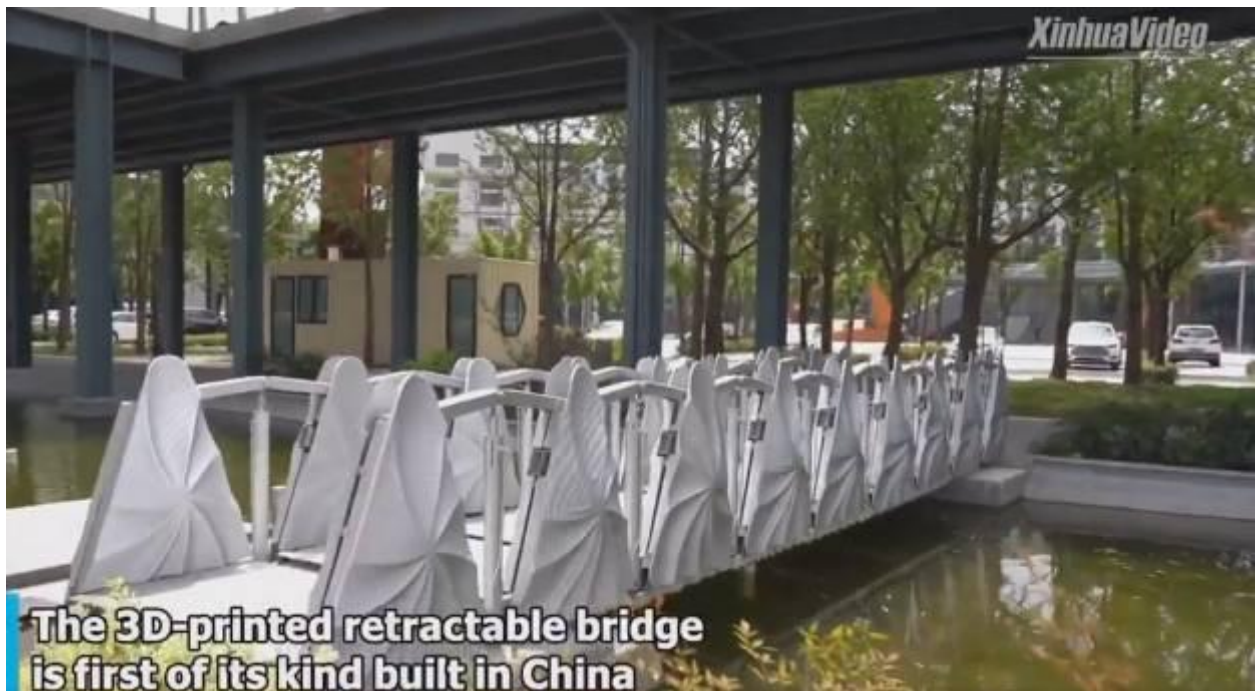
Pic. 2: A swing bridge built with 3DP in China.
