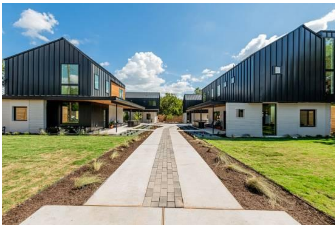
Pic. 3: General view of houses, ground floor created with 3DP in the USA.
